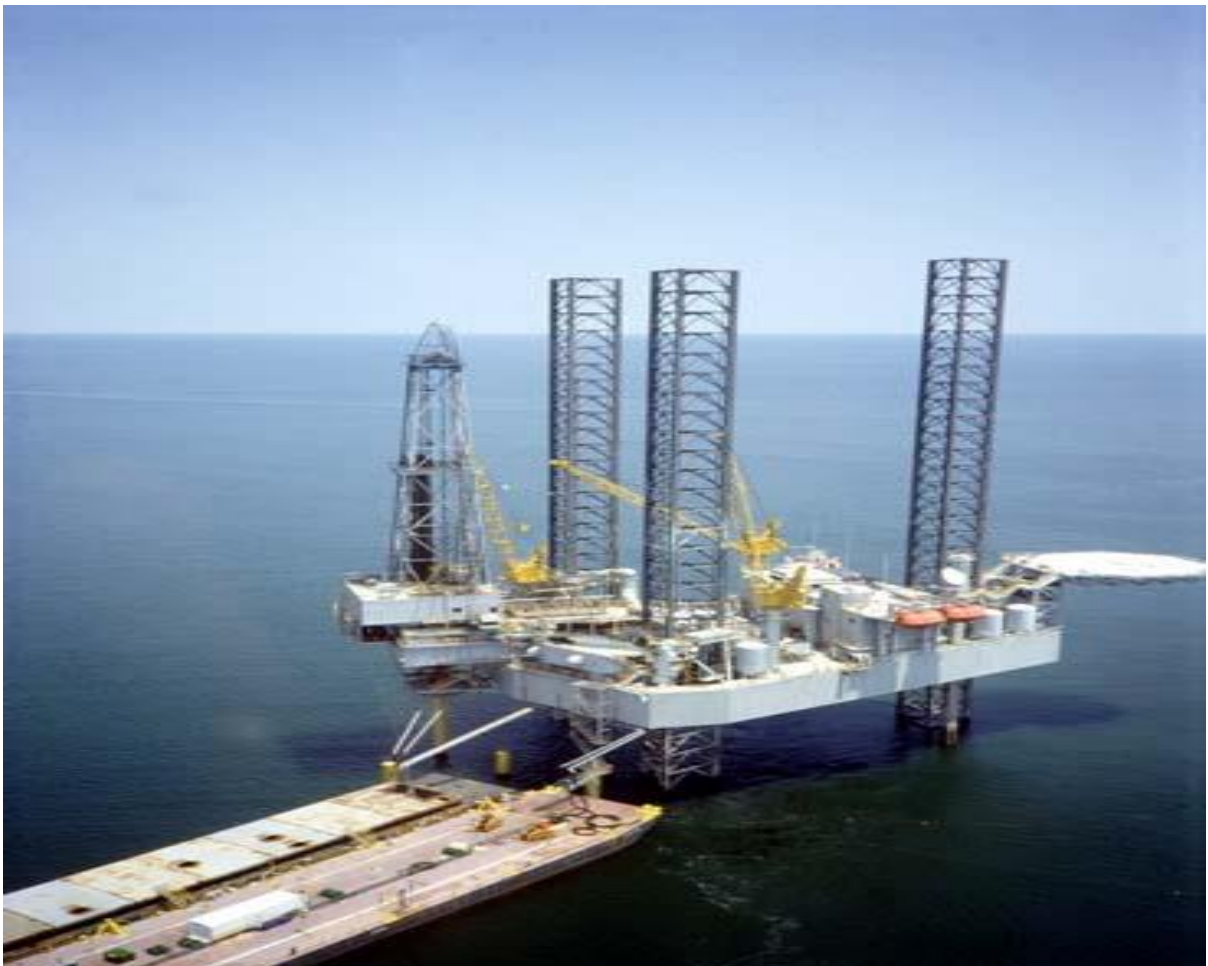
Figure 11. Offshore production platform.
