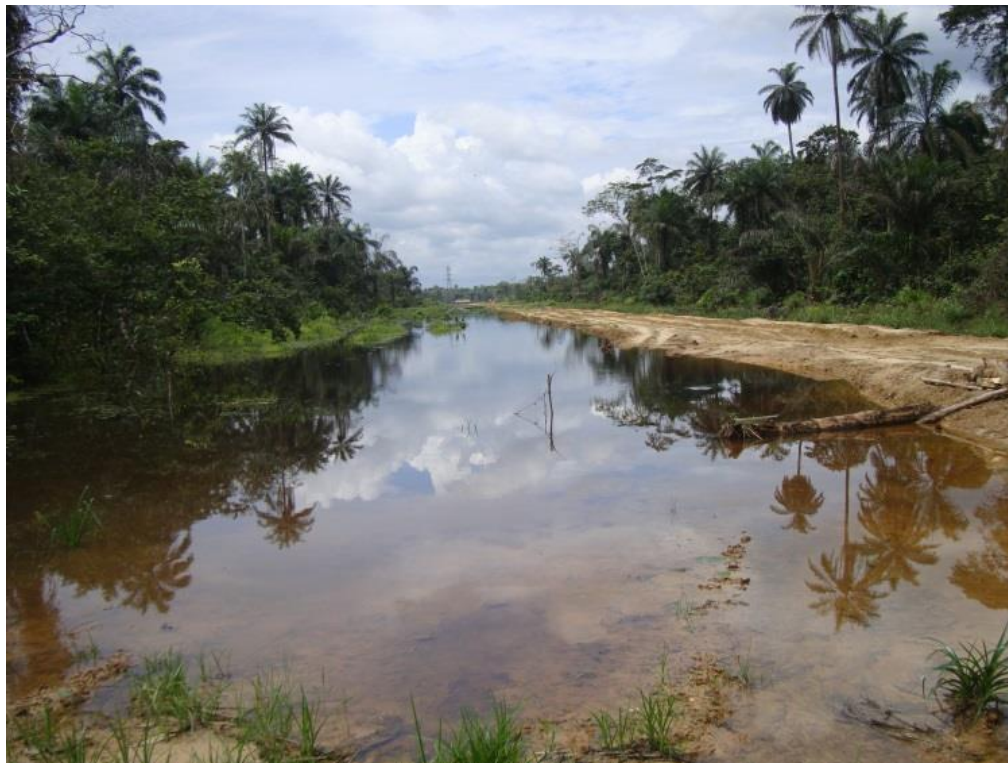
Figure 15. Buried oil pipelines.
